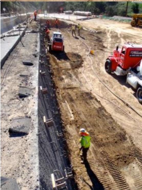
Crews are stabilizing the cut banks with gunite, a sprayed on cement.
