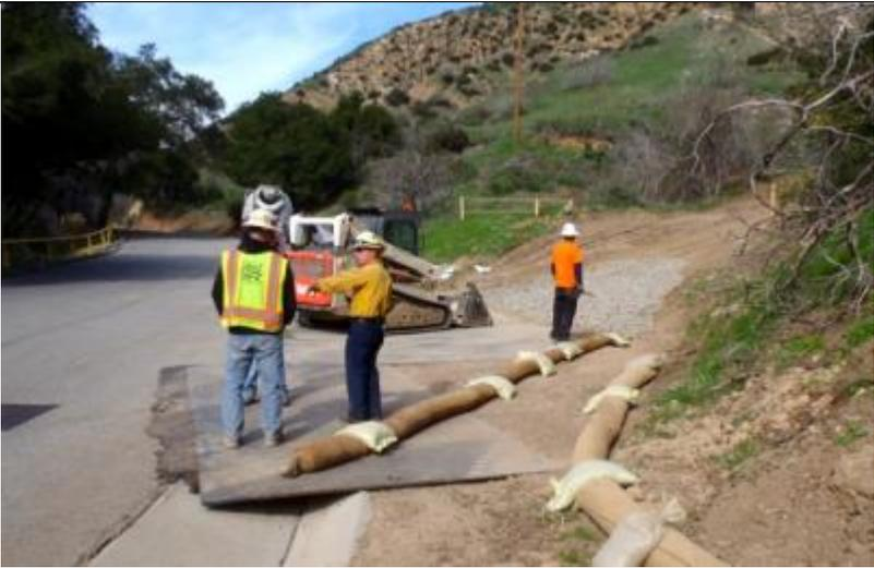
A photograph showing three construction workers in safety gear on a road. The road surface is being prepared with gravel and steel plates. A small orange utility vehicle is visible in the background. The road is bordered by a dirt embankment and some trees.                                             | The TSP 46 access road is being prepared with gravel and steel plates where it meets the main road. |
